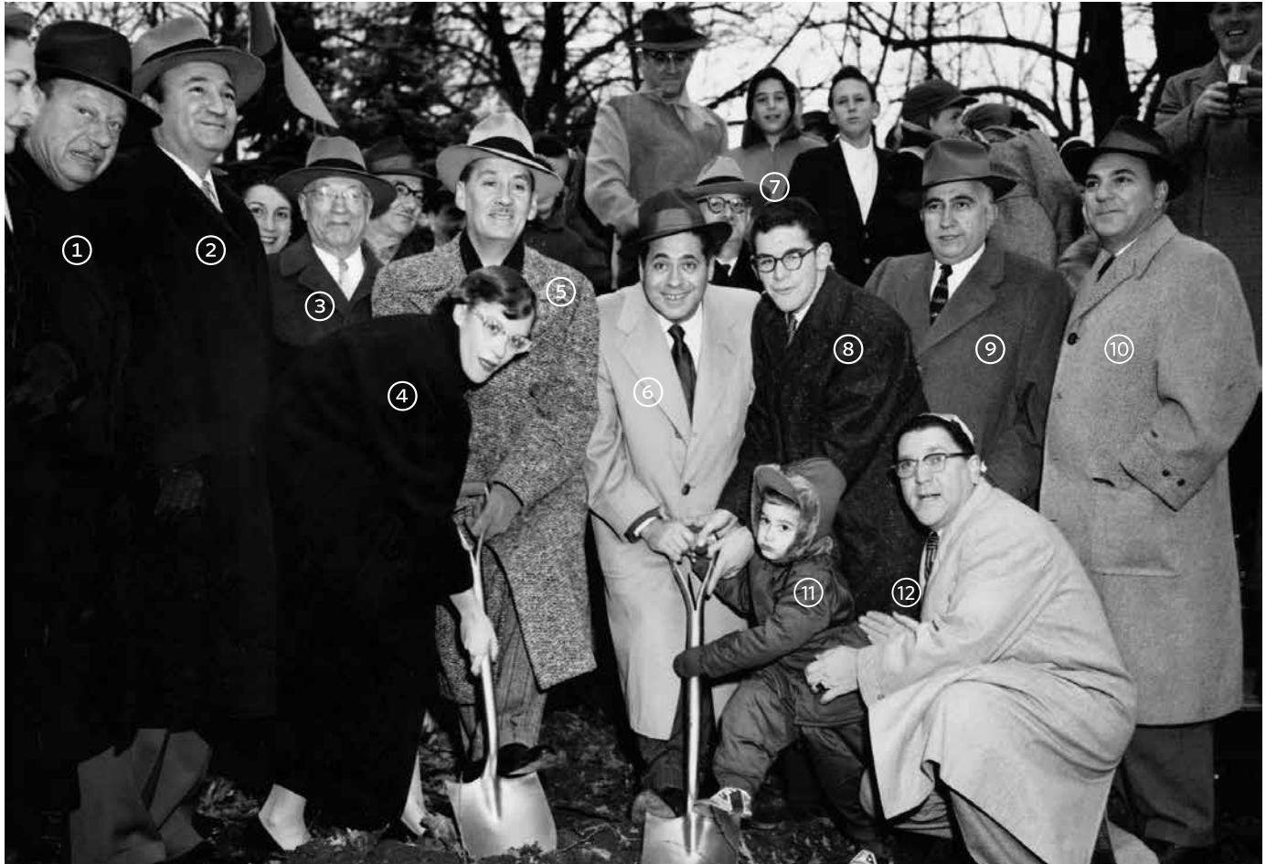
Groundbreaking for the "Community Center" (Auditorium) – November 27, 1955
